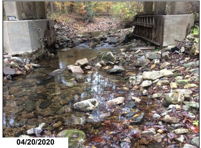
Bents 2 & 3 bottom of footing exposed on channel side of bents.
