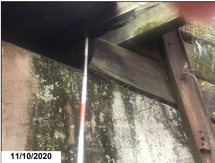
Cribbing decay in timber abutment at bent 4 right side.
