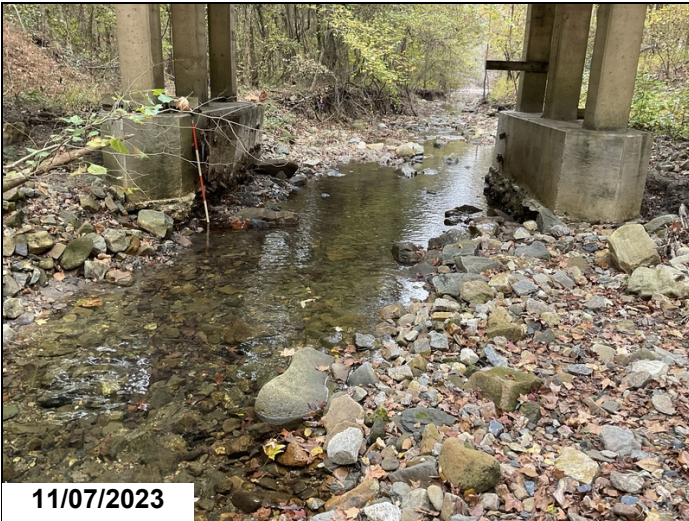
Bents 2&3: both footings are exposed due to scour action. 2023
