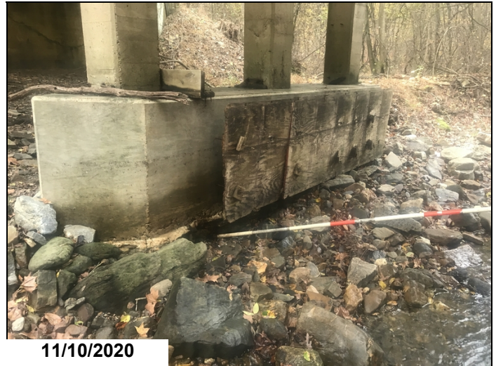
Back side bent 3 footing is exposed.
