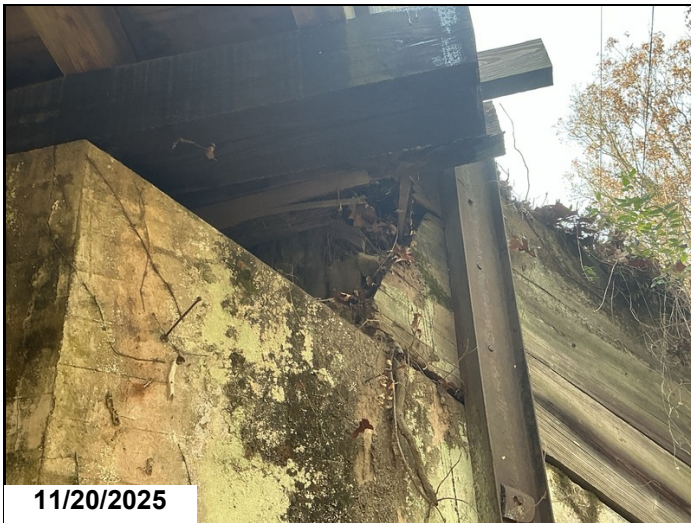
Cribbing decay in timber abutment at bent 1 left side. 2025
