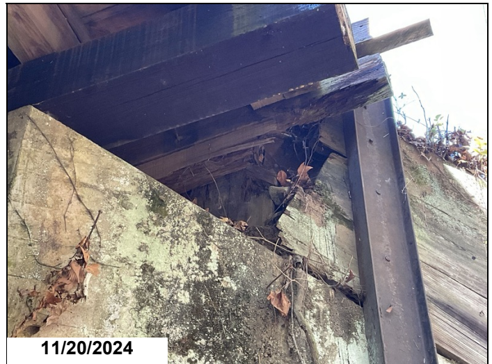
Cribbing decay in timber abutment at bent 1 left side. 2024
