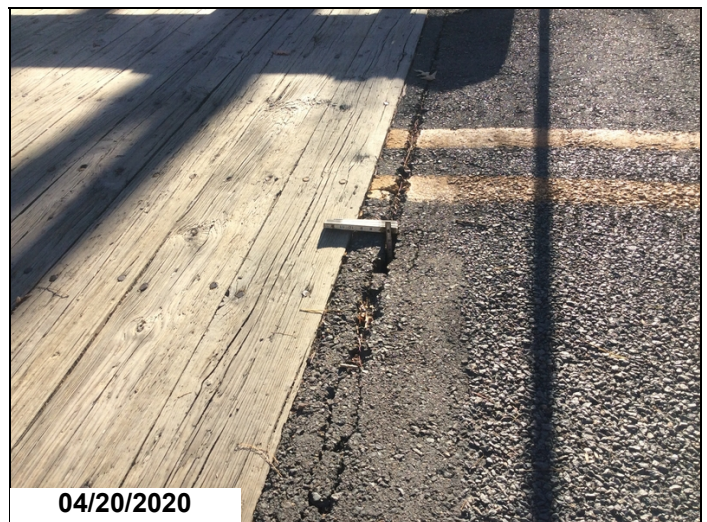
Bent 1, void in the approach.
