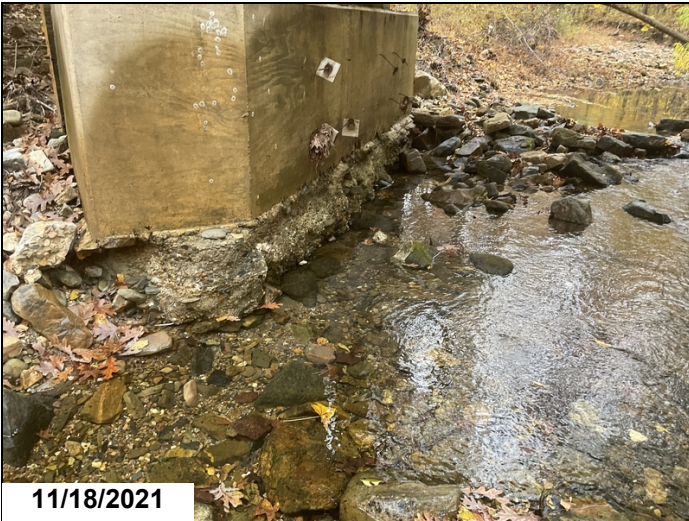
Bent 2 footing ahead bottom of footing exposed.
