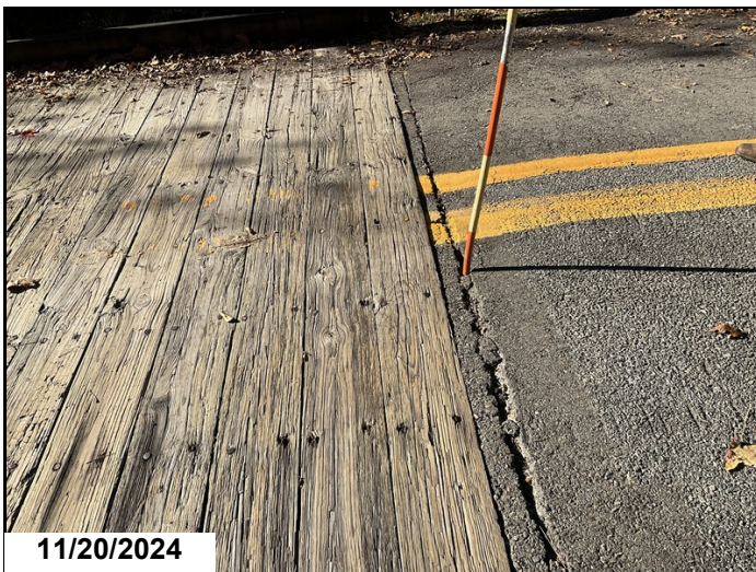
Approach roadway north end of bridge small void in the road at bridge end due to cribbing decay. 2024
