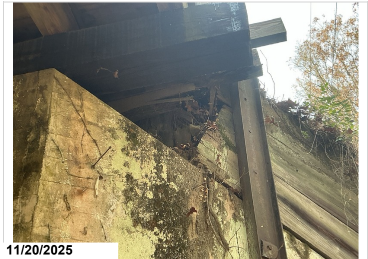
Cribbing decay in timber abutment at bent 1 left side. 2025
