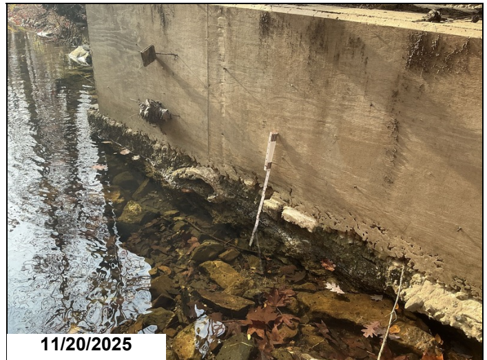
Ahead side of bent 2: footing is exposed.
