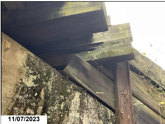
Cribbing decay in timber abutment at bent 4 right side. 2023
