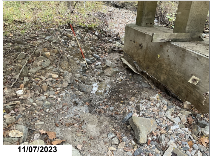
Bent 2: backside of footing is exposed due to local scour action. 2023
