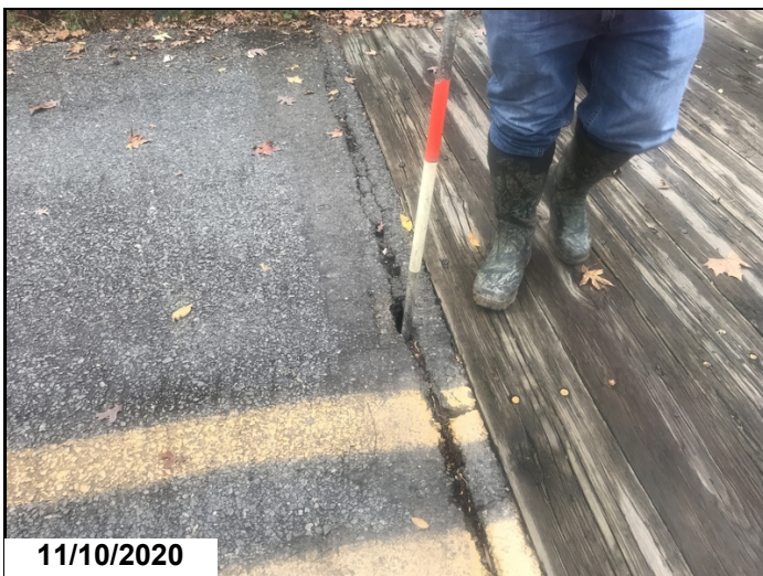
Approach roadway north end of bridge small void in the road at bridge end due to cribbing decay.
