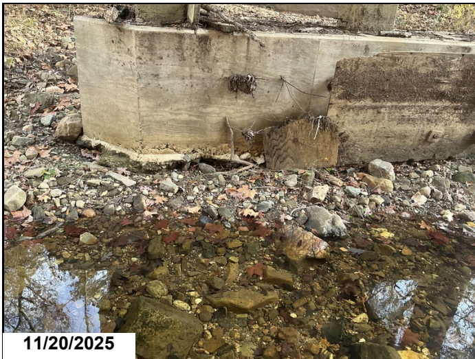
Bent 3: footing is exposed.
