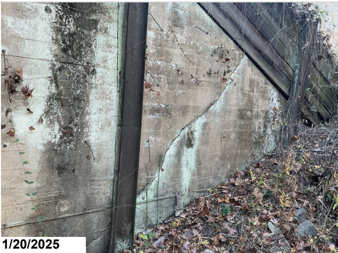
Bent 1: left side of abutment the wingwall with large diagonal cracking
