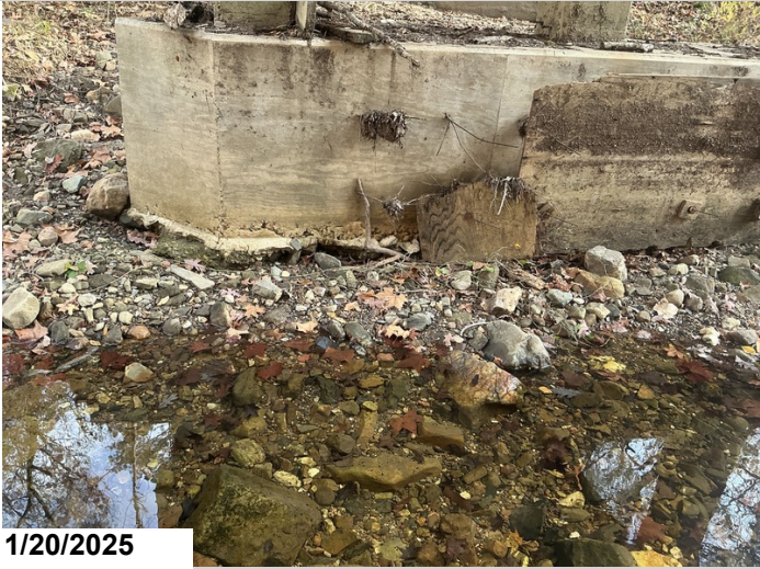
Bent 3: footing is exposed.
