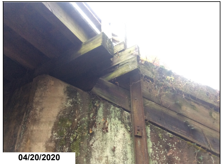
Bt. 4 timber cribbing has decay.
