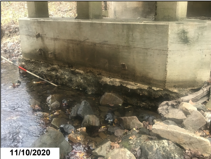
Bent 2 ahead side of footing is exposed due to scour.
