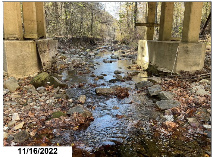
Looking at both bents 2 and 3: both bottom of their footings are exposed. 2022
