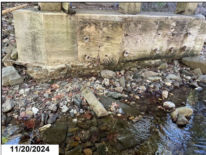
Bent 3: Scour action has exposed the footing. 2024
