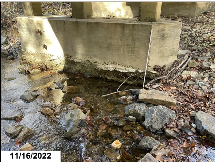
Bent 2: Scour action has exposed the footing and has some undermining. 2022
