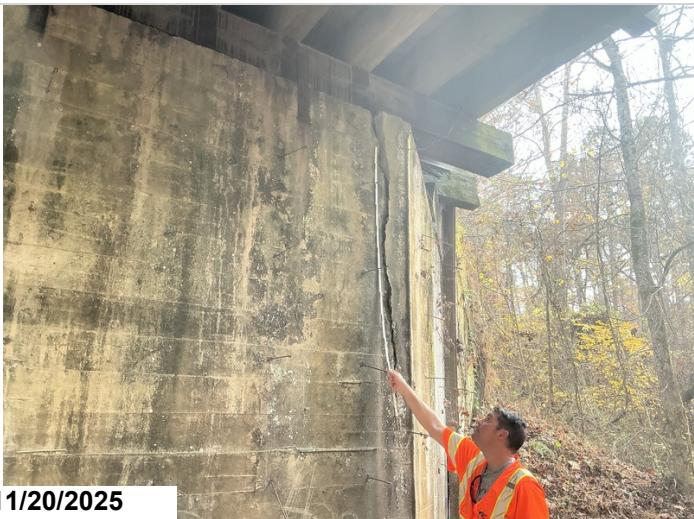
Bent 4: Large vertical crack on the right side of the abutment that is separating.
