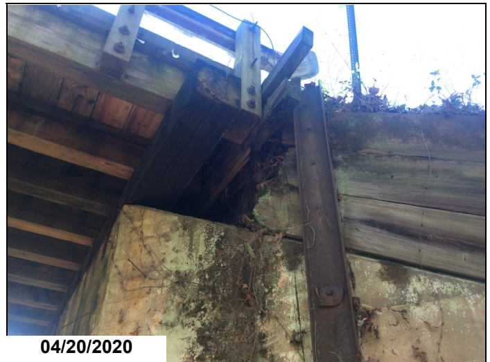
Bent 1, decayed timber cribbing.
