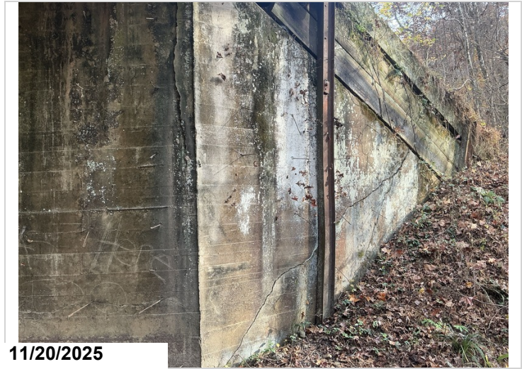
Bent 4: cracking in the wingwall.
