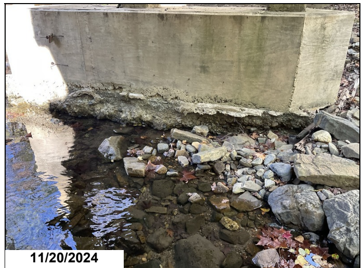
Bent 2: Scour action has exposed the footing. 2024
