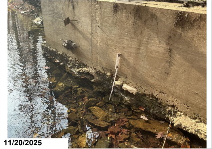
Ahead side of bent 2: footing is exposed.
