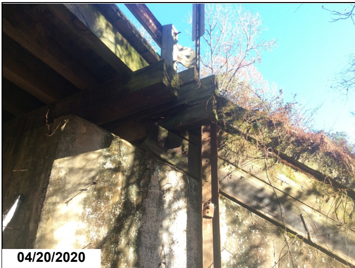
Right side of bent 4 cribbing decayed.
